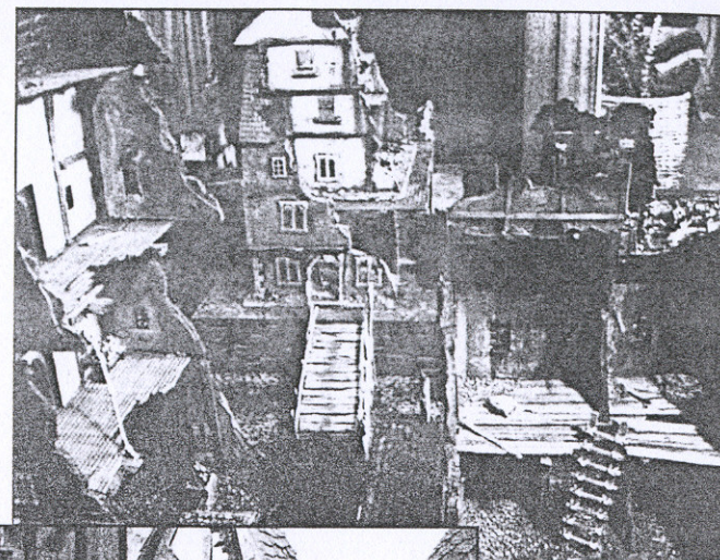
Another view showing the wooden walkway and several ruined buildings.
